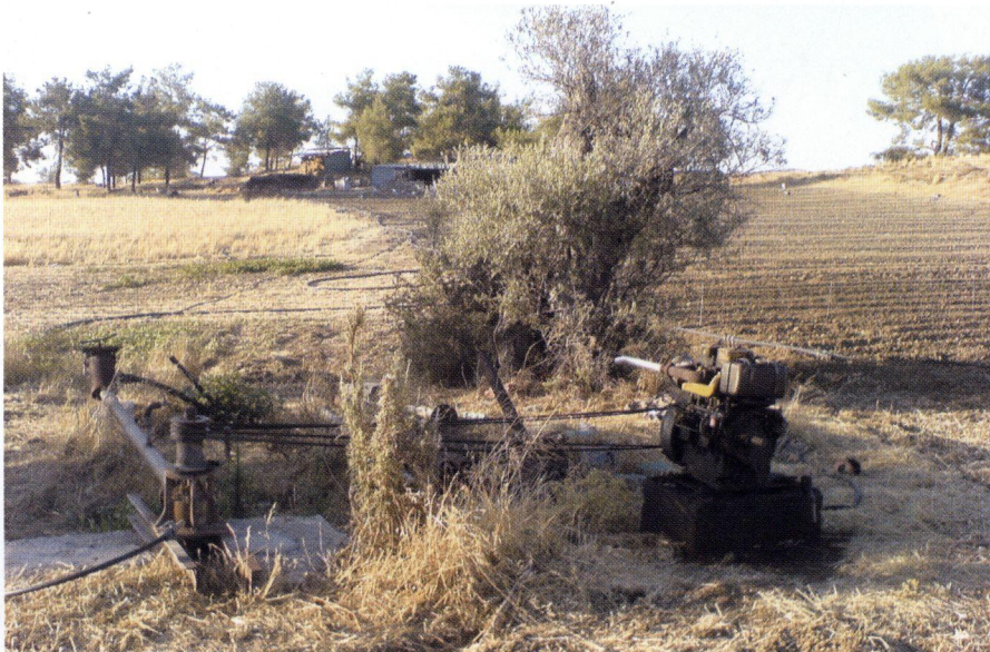
b: One of the many still active diesel pumps for irrigation. Sia-Mathiatis area.
